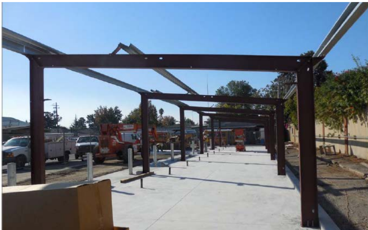
Steel Framing for New Corporation Yard Storage Building
