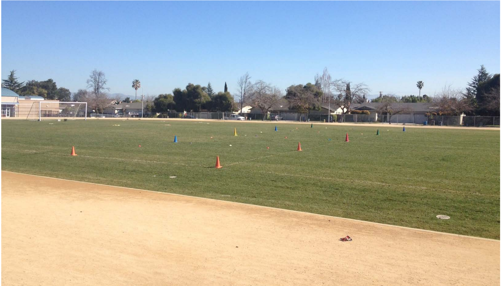
New Track and Field Lawson Middle School
