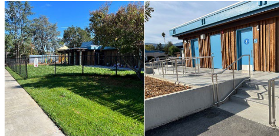
Kindergarten Yard Expansion & ADA Improvements
