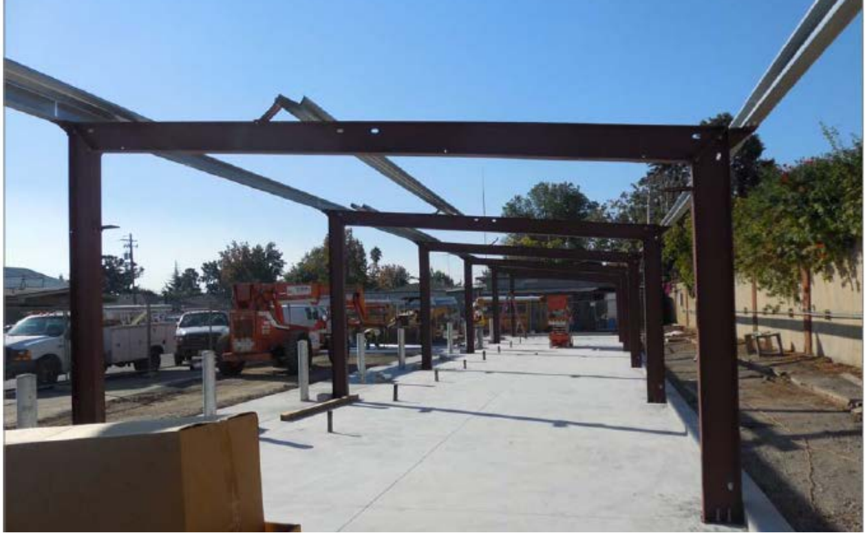
Steel Framing for New Corporation Yard Storage Building
